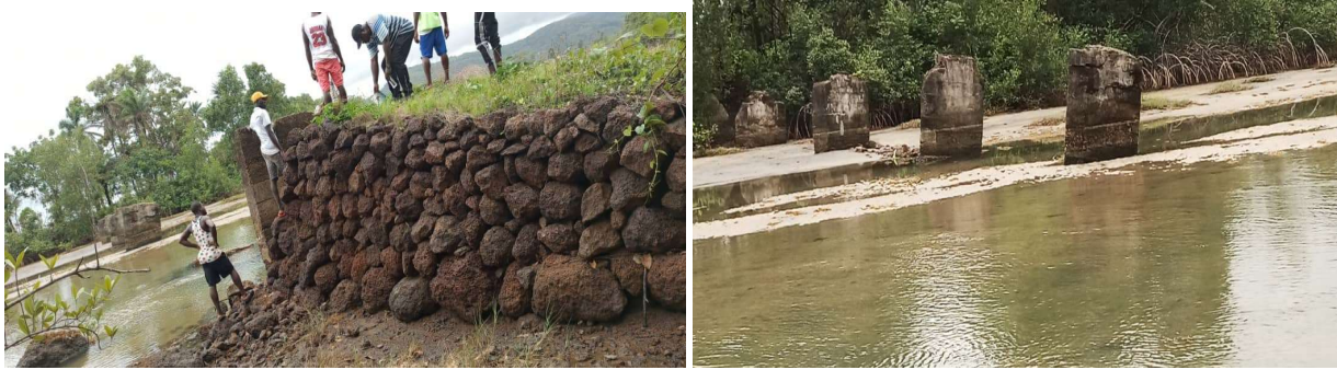
Figure 41. Flood Inundation of Mangroves, Breakwater, and Bridge at Black Johnson Lagoon
