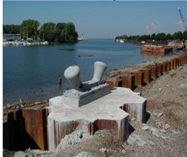
B) Bulkhead foundation backfilling
