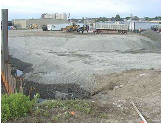
C). Backfilling for Dewatering
