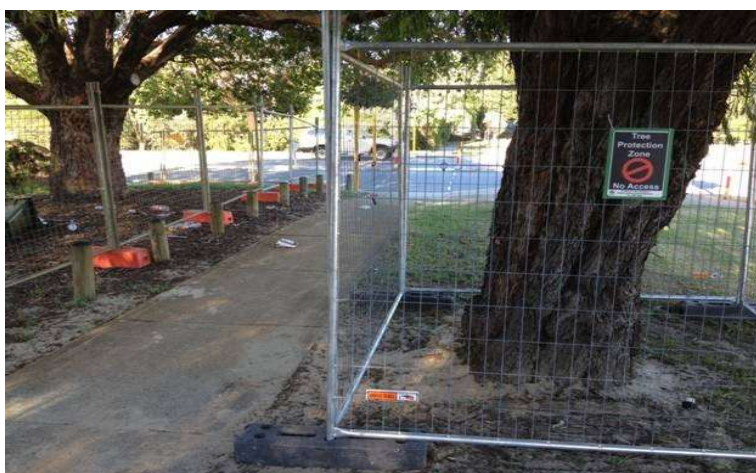
Figure 49. Typical Verge Street Tree Protection Barricade with Signage
