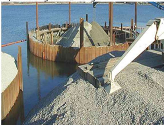
C). Backfilling for Dewatering
