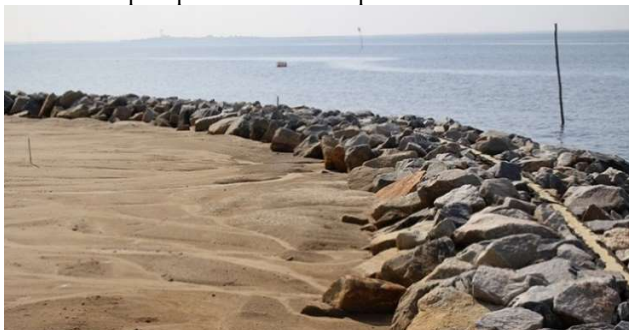
E. Rock -Rip Rap Breakwater Proposed
